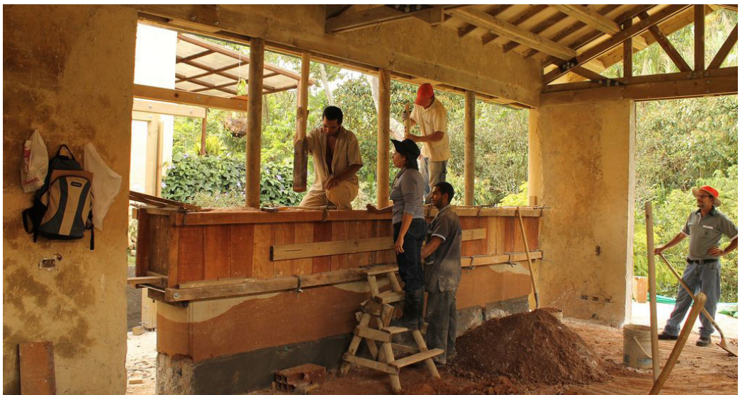
Figure 5. Workers of "tapia pisada" in Colombia. Source: Escala Urbana Arquitectura, Casa Mila project
