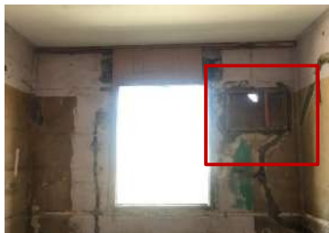
(Fig.64) - Installation of one unit cooling system. Source: Author
