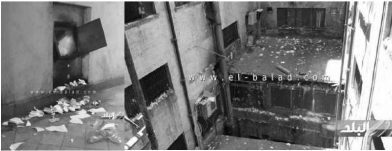
(Fig.43) - Internal photos from the building. Source: Al-Nagar, 2016)
