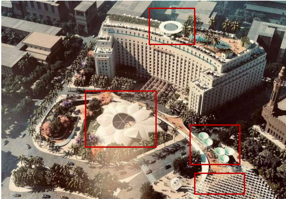
(Fig.51) - Proposed new function design for the building. Source: The American organization (Oxford capital group) edited by the author
