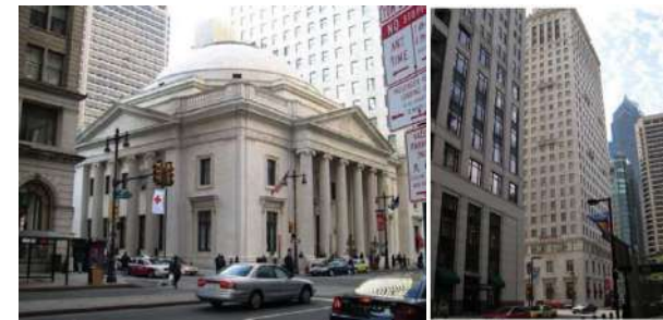
(Fig.37) - Dome and tower building, Source: (Catherine, 2005)
