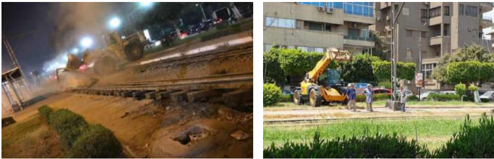
Figure 38: Removing the tram line in Heliopolis – Source: Facebook group (HHI , 2019)
