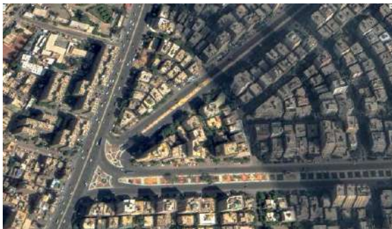
Figure 52: The intersection between Gesr al Suez, Abd el Aziz Fahmy and Mohamed Farid streets in 2021 after the development – Source: Google earth satellite images
