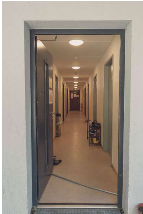
Figure (4.26) Main Door Kept Open Using a Metal Rod Source: Author
