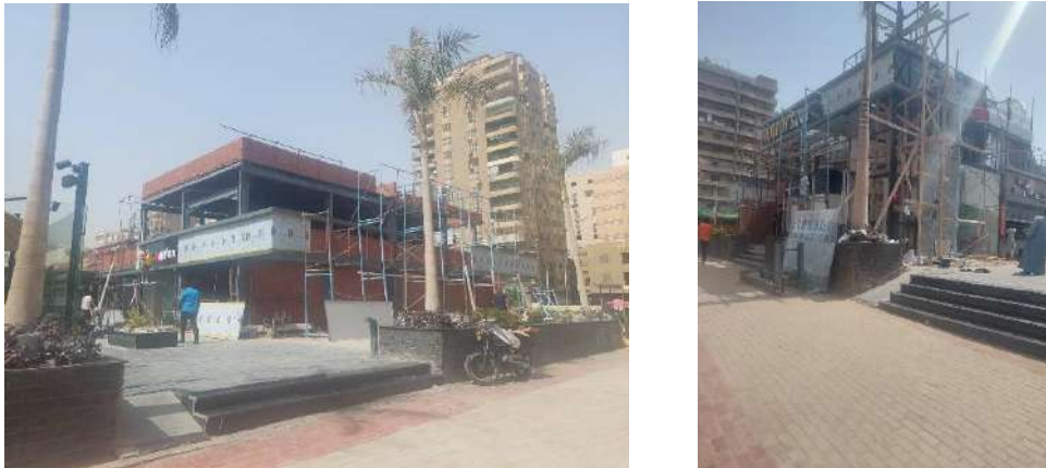
Figure 67 :shows the structure of one's of the commercial building using steel beam and high percentage of solid wall in contrary of the government unofficial requirements of using glass.
