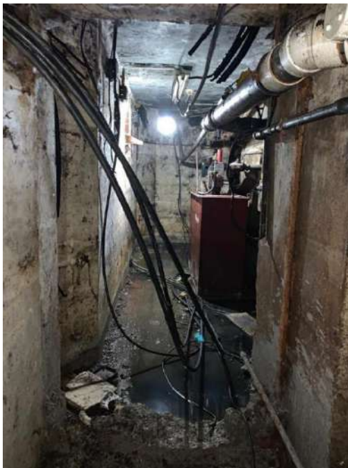
Figure 49 Basement water sedimentation (Source: Ahmed Mady)
