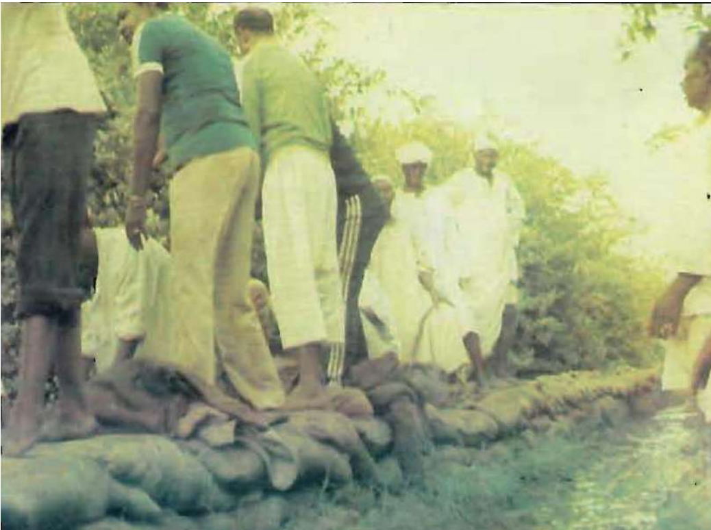
Figure 47- Building the barrier with sand sacks- Tuti 1988. Source: Mr. Hafiz Mohamed.
