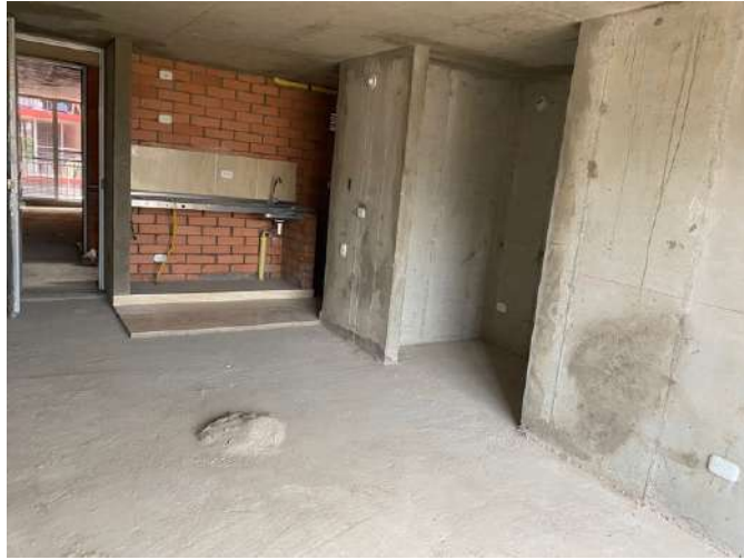
Figure 8: Kitchen inside Social Housing Unit
