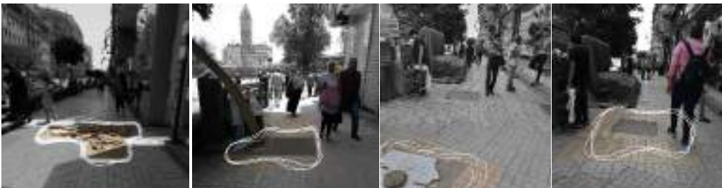
Figure.87- Sidewalks deterioration at 26 July street. Source: Researcher.
