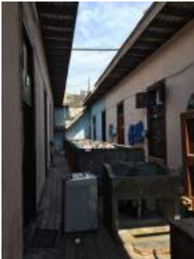
Figure 36: Second floor in 'El Arca'. Source: the author.
