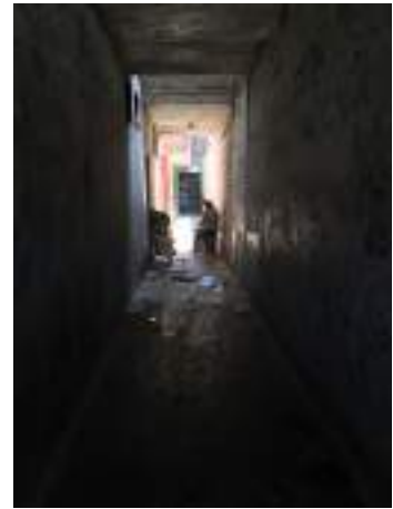
Figure 26: Shared roofed access corridor in horizontal housing building. Source: the author.
