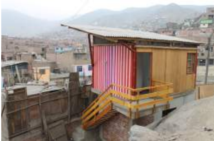
Figure 11: The housing module built by IVUC and PIH. Source: IVUC, 2015.
