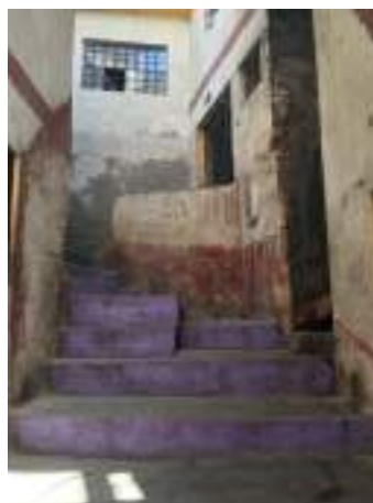
Figure 27: Alley and stairs inside CSC. Source: the author.
