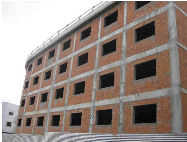
Figure 7: Concrete skeleton building
