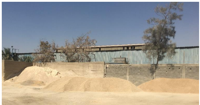
Figure 20: Piles of sand and gravel to be mixed manually to form concrete. (Source: The author)
