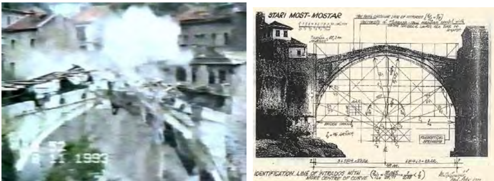
(fig. 45)— Left image: destruction of the bridge on 9th of November 1993.
