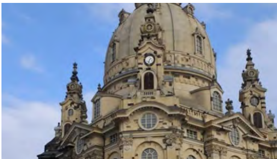
(fig. 18)— Photo of the Frauenkirche. frauenkirche-dresden.de (2017): under the guiding principles of reconstruction: “The dark coloring of the old stones and the dimensional differences in the joint areas between the new and old masonry resemble the scars of healed wounds.” Source: Author (2017)
