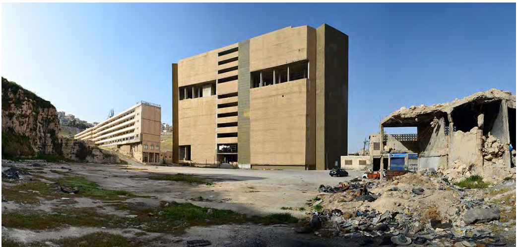
Figure 40 Main entrance (Aljabi 2016)
