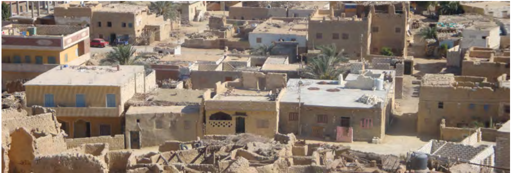
Fig.35:a group of four modern structures using concrete roofs, source: author, 2016.
