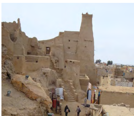
Fig.68: Photos of two main mosques in the focus study area, top: westerners mosque, bottom: ancient mosque of Shali, source: author, 2015.
