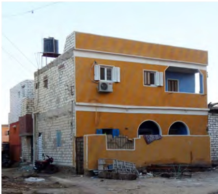
Fig.36:A modern structure with bright facade colors, source: author, 2016.
