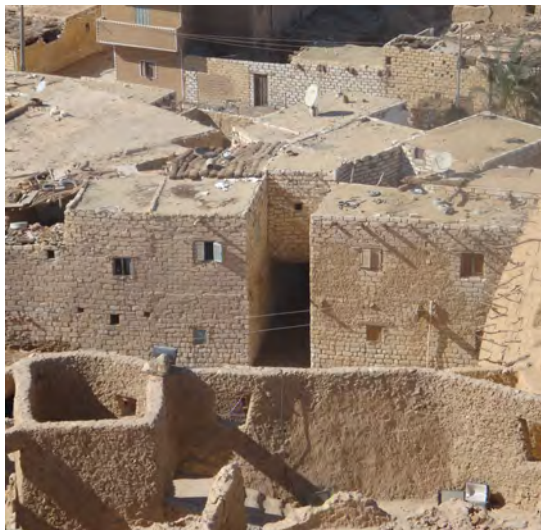
Fig.34: a mixed structure house rebuilt using stone bricks, source: author, 2016.
