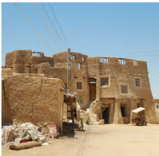
Fig.31: new-vernacular house with a khoss turned into a private loggia in the ground floor, source: author, 2016.
