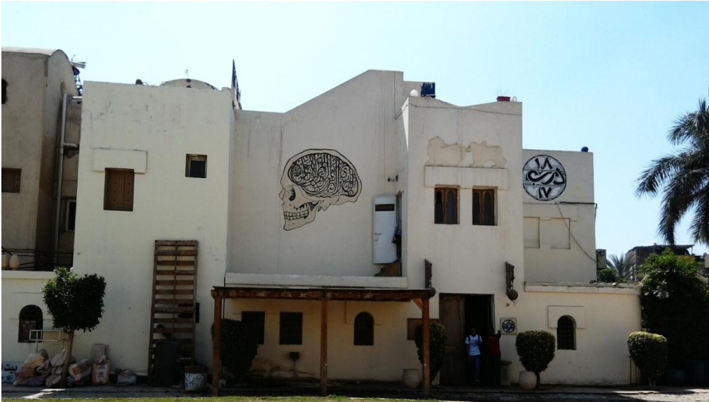
Figure 28: Darb 1718 main building
