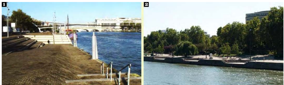
Figure.66: Renovated dike-profile next to the National Library in Paris.
