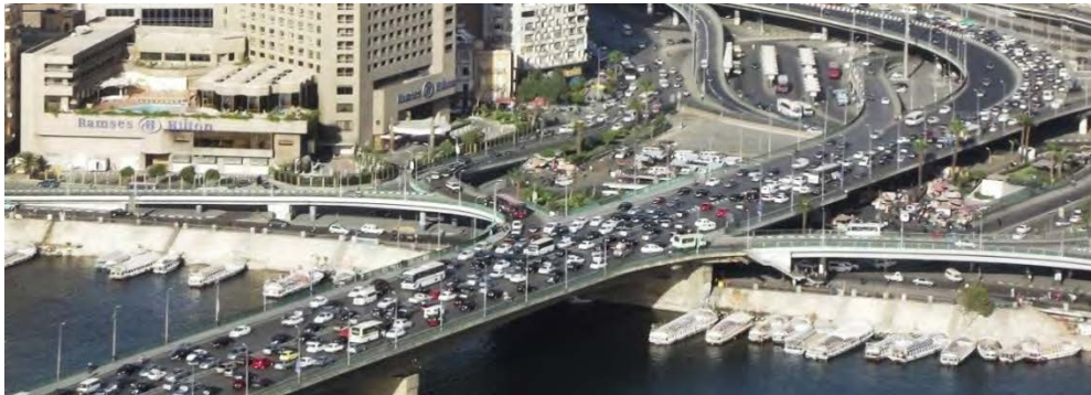
Figure.37: Massive traffic jam in Abdel-Moneim Riyad square connected with 6 th of October Bridge. Source: Author.
