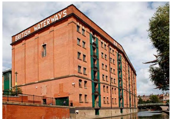
Figure.6: Rehabilitated Warehouse in Nottingham Canal, UK. Source: Zabulis, 2013
