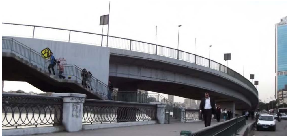
Figure.39: 15 th of May Bridge blocking the river view. Source: Author.
