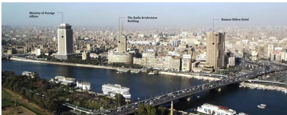
Figure.26: Panoramic view shows the main buildings- east bank in sector 2. Source: Author.
