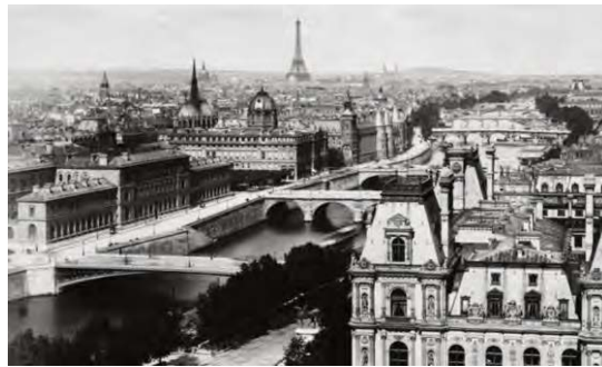
Figure.61: Flood protection wall in 1900.
