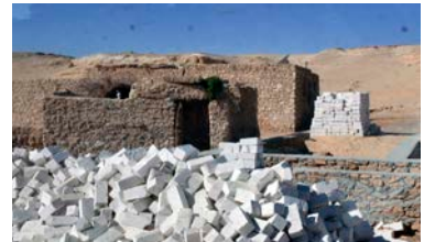
Figure 6.62: Building with the Limestone bricks is being emerged in The Village 's architectural style
