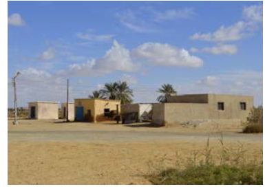
Figure 5.17: The diesel power-generating unit
