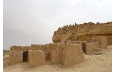
Figure 6.03: An abandoned vernacular house in The Village
