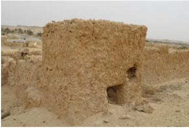
Figure 4.29: The hūr with a southern outlet opening
