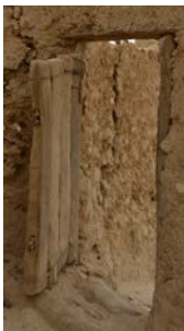
Figure 6.11: An old door made out of palm tree trunks
