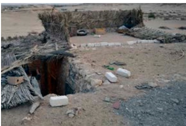
Figure 7.16: Roofs are just covered with plastic sheet and earth layer
