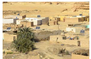
Figure 5.18: Houses are provided with PV units
