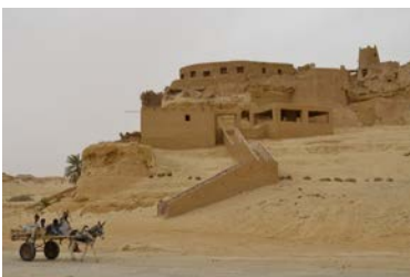
Figure 5.16: The rehabilitated part of the Old Şālī
