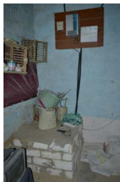
Figure 6.33: PV interior corner
