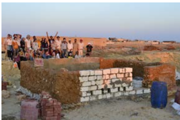
Figure 3.09: The 4 x 3 m 2 room constructed during the Siwa Spring School (May 2013)
