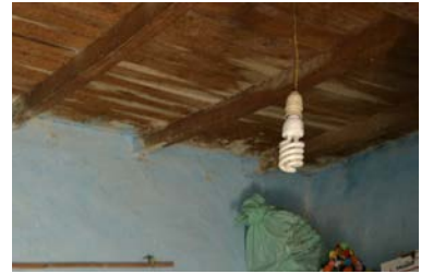
Figure 6.15: Wooden panels are used for roofing in the original prototype structure
