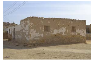
Figure 6.12: Sample house unit of 'Allām Housings
