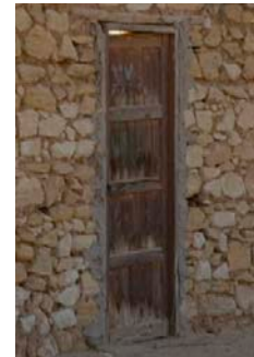
Figure 6.17: Sample entrance door in 'Allām Housings private entrance
