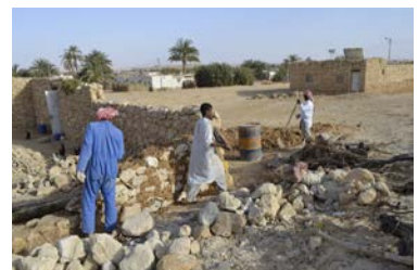
Figure 3.07: The master builder and two assistance during the interview on-site
