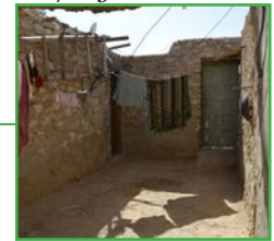
Figure 6.55: Another internal courtyard
