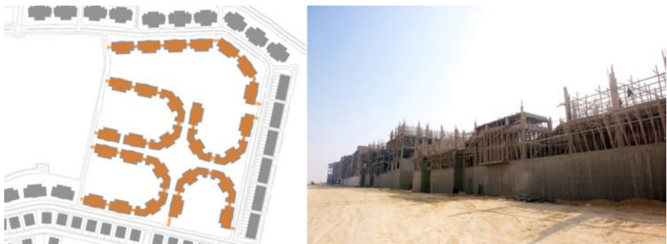
Figure 53: Underground car parking in NewGiza Left: The colour represents the underground car parking's that are connected via underground tunnels. Right: Massive concrete construction needed for such tunnels. . Source: Author as adapted from (Earth, 2008)..
