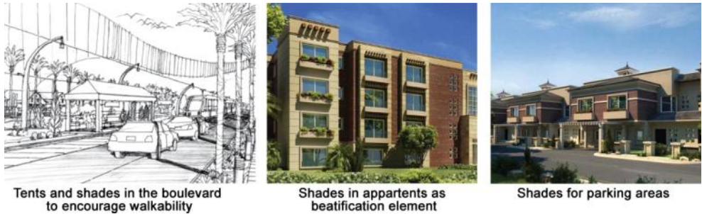
Figure 55 External shades in NewGiza. Source: (Earth, 2008). (NewGiza, 2011)
