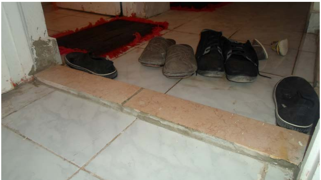
Many Syrian families mentioned installing this pavement at door-steps to help in cleaning each room with water
