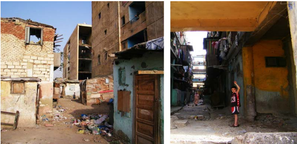
Figure 5-13: Left: Tobgeya housing blocks before demolishing illegal units in 2010. Right: deteriorated conditions of block number 3 in Tobgeya (Source: author).
