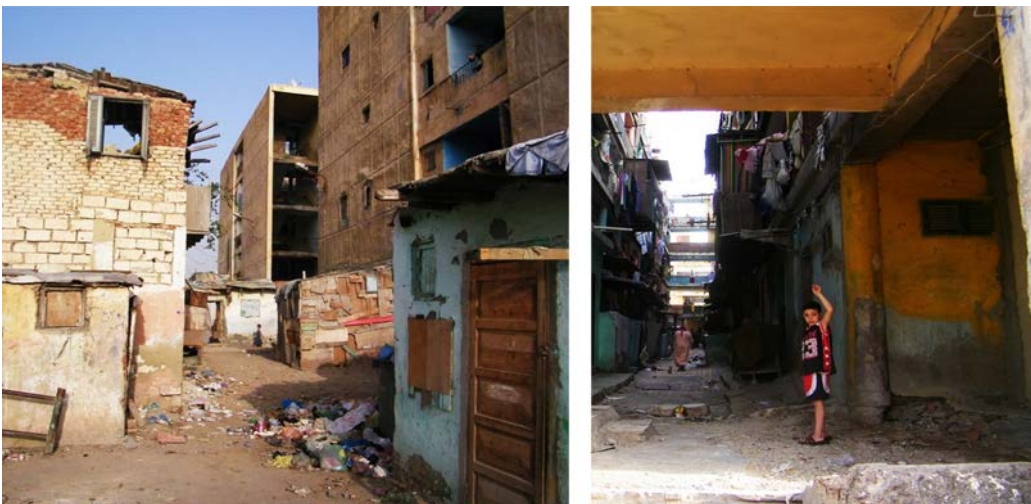
Figure 5-13: Left: Tobgeya housing blocks before demolishing illegal units in 2010. Right: deteriorated conditions of block number 3 in Tobgeya (Source: author).
