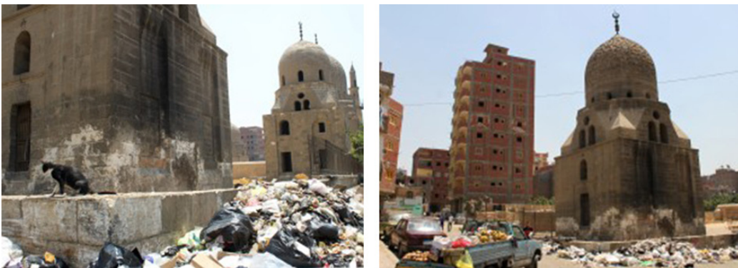
Figure 4-3: Badly damaged 15th-century mausoleums are now surrounded by growing piles of trash in the Manshiet Nasser slum. Illegal high rise buildings appear in the background (source: Jones, 2014)
